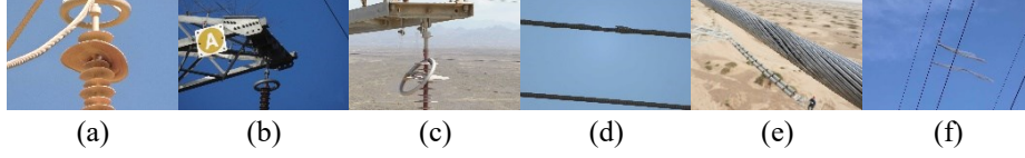
Fig. 1. (a)insulator damage, (b)grading ring tilt, (c)grading ring abscission, (d)cable strand disconnect, (e)cable loose strand, (f)cable foreign object.
