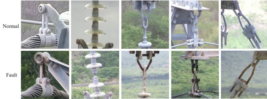
Fig. 1. Sample images of InsPLAD, including normal and fault conditions.
